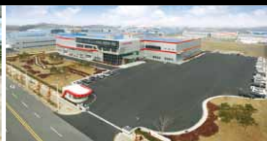
● SAMICK THK CO., LTD. DALSEONG PLANT (KOREA) Site: 34,886m 2 (375,118sq.ft.) / Floor space: 8,324m 2 (89,505sq.ft.)
