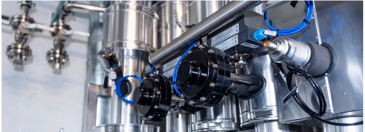
Space-saving Schubert & Salzer sliding gate valves in the tight-fitting Bachem AG plant.
